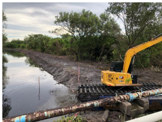
Fig. 14: Dredging carried out by Department of Irrigation & Drainage, DID at Sungai Lutong to deepen the channel
