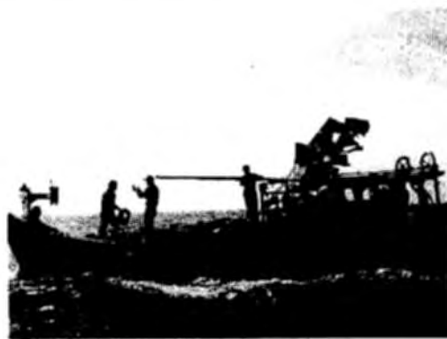
Fig. 5 FED installation by local fishing boat.
