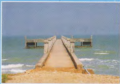
The pier made of concrete was constructed by the DOF.
