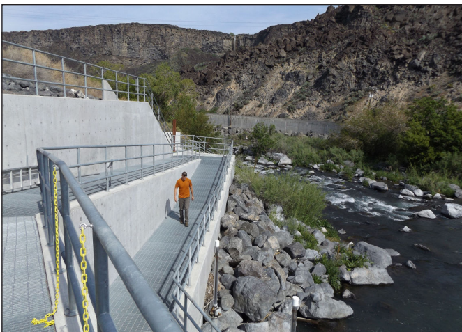
"Senior fisheries biologist for Idaho Power, walks down the fish ladder beside the diversion dam for the utility's Lower Malad hydroelectric plant May 13. Below the grate at his feet, fish can swim up or down the ladder through a series of pools."
