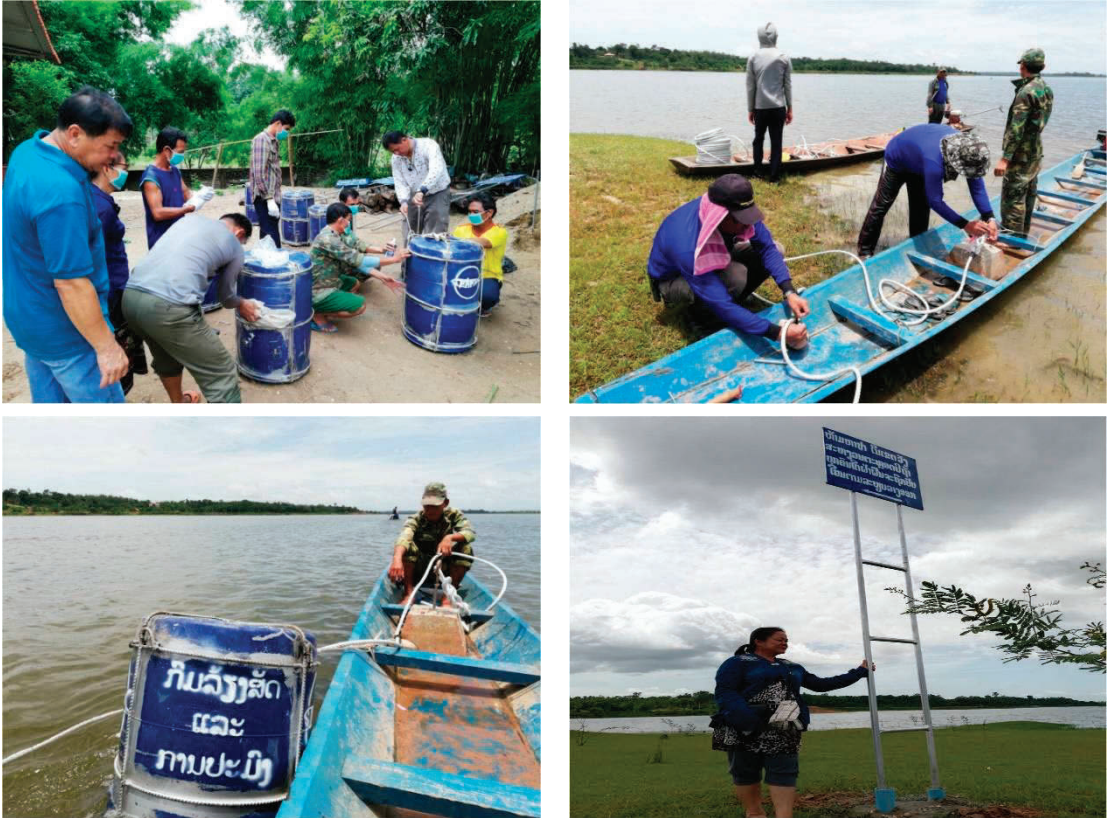
Fig. 100-103 Installation of buoys and sign boards at PH District
