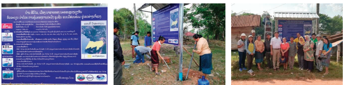
Fig. 80-82 Installation of the four (4) big signboards at Naxaythong District
