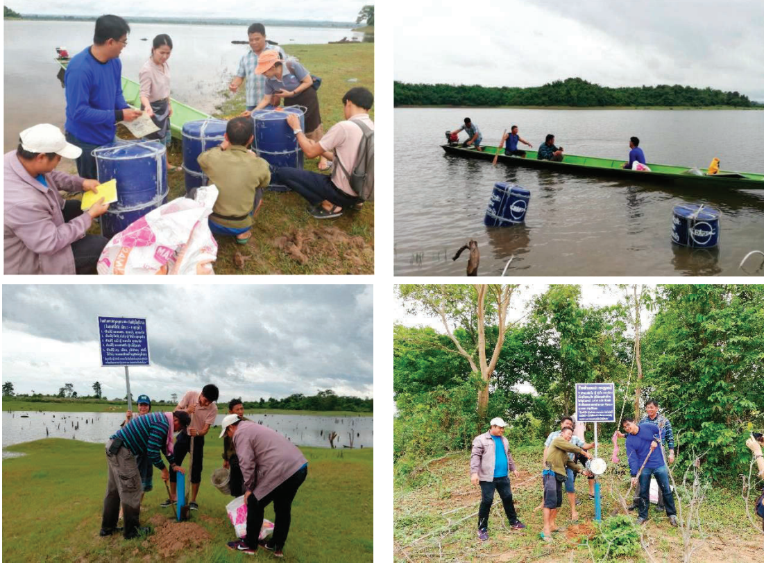
Fig. 104-107 Installation of buoys and sign boards at NT District
