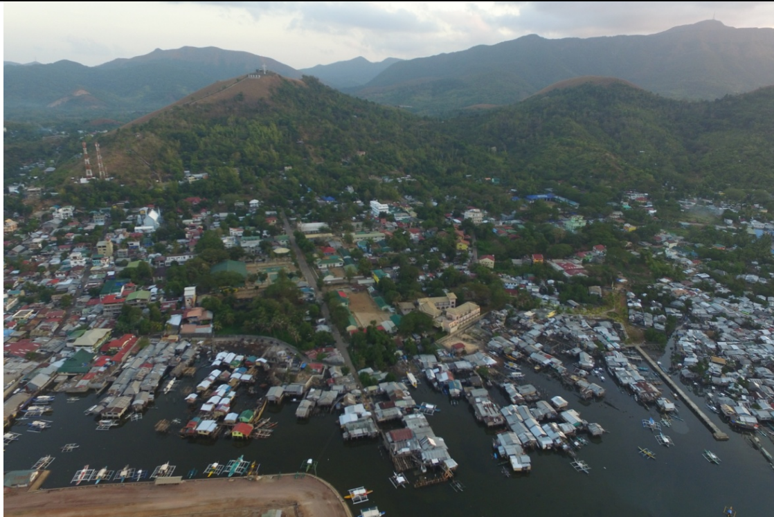
Aerial Photo of Coron Town
