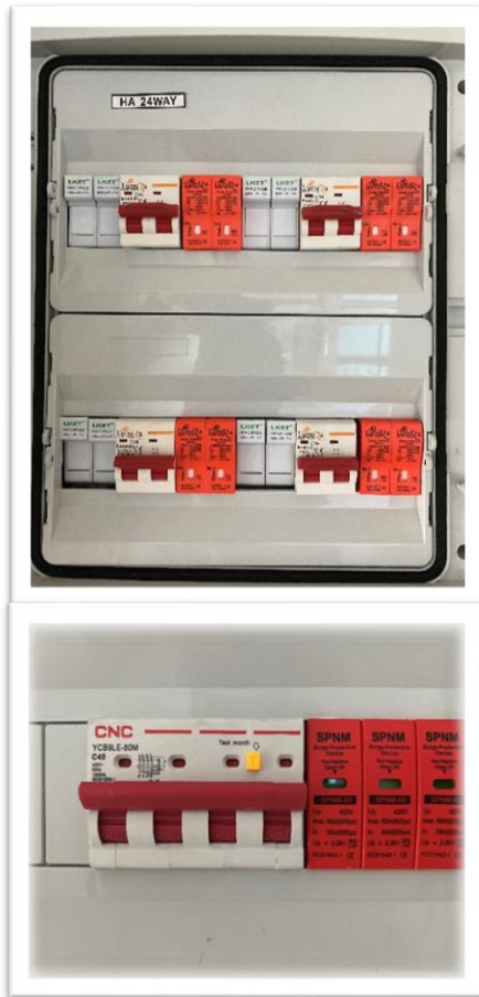
Illustrate 11. DC/AC circuit breaker
