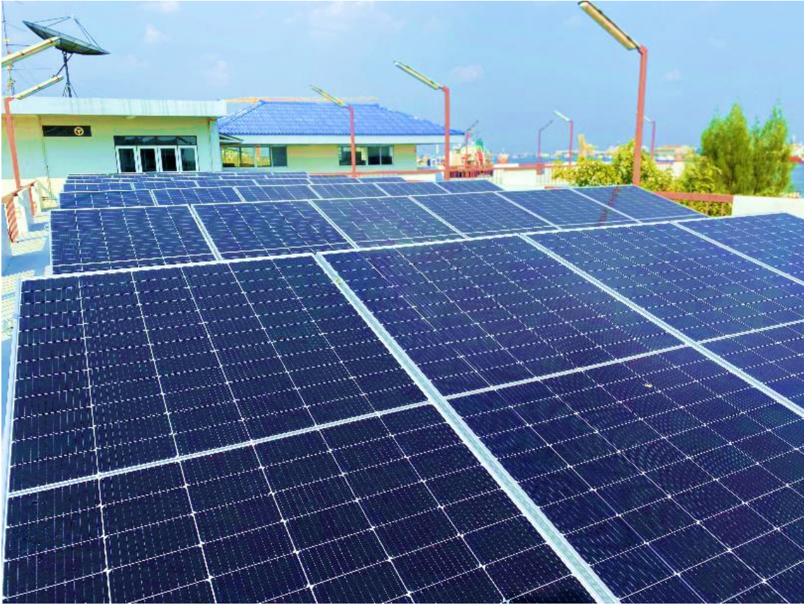
Illustrate 2. On-grid solar roof system for Training Department
