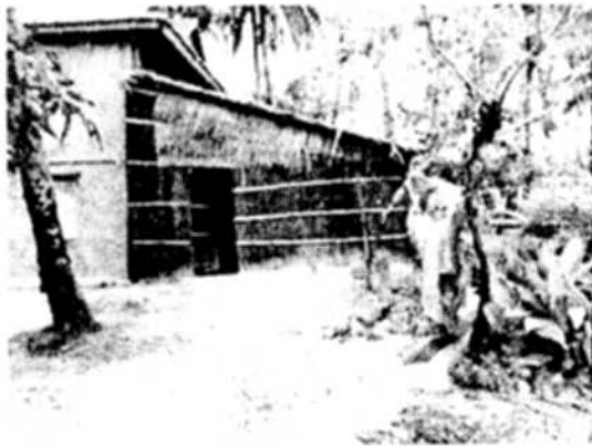
Newly constructed mushroom storing yard
