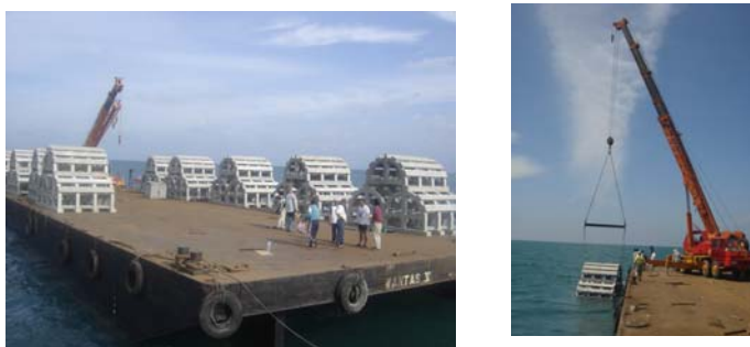
Figure 5. Installation of ARs by LKIM on 20-22 January 2006
