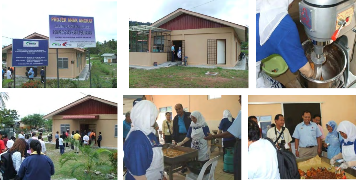
The newly constructed fish processing plant for the KEW: construction and equipping with modern facilities was done through the DOF Malaysia
