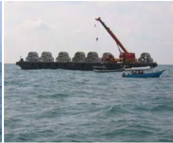
ARs properly stacked and loaded at both sides of the barge
