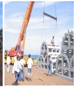
ARs ready to be installed at identified position
