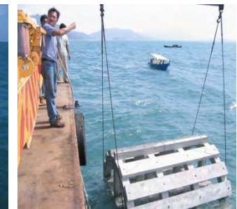
ARs unloaded and placed on the seabed
