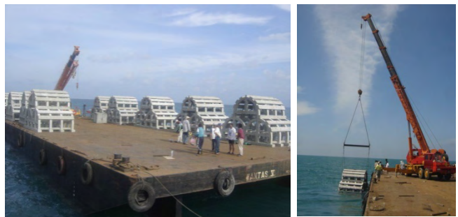
Fig. 31. Installation of ARs by LKIM on 20-22 January 2006
