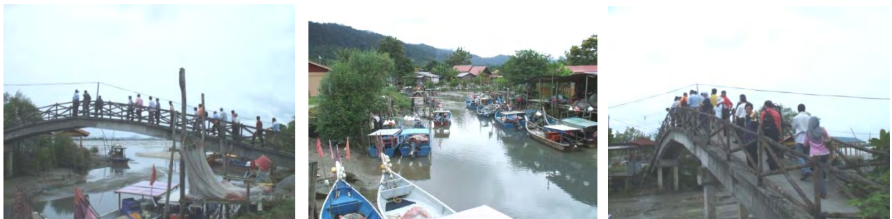
Access bridge over the canal in Kuala Teriang (a post-tsunami infrastructure)
