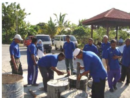
Fig. 6. Preparation of cement anchors
