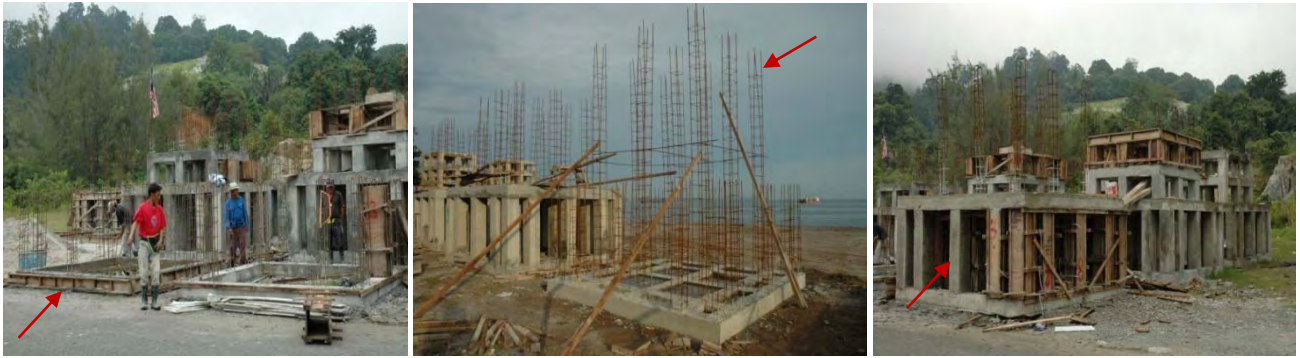
For soft-bottom ARs: construction of base (left), construction of solid steel bar 1.2 cm dia (center), and construction of 25 piles (right)
