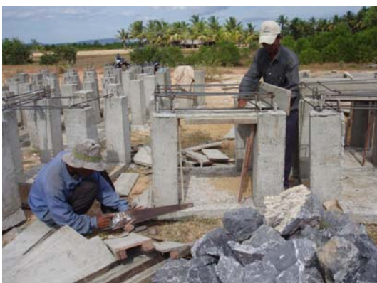
Pic 1: Construction of obstacle objects
