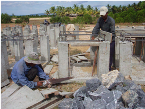
Fig 5 Construction of obstacle objectives
