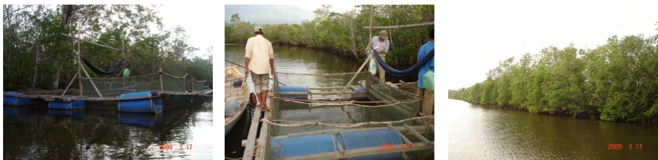
Fig. 2 Fish cage construction at canal in Kampong Chin village
