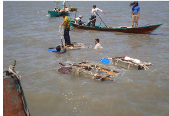
Fig 6 Installation of obstacle objectives
