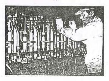
67. It is not always possible to rely solely on instruments to detect engine trouble even given the present advanced state of technology. A good engineer must also cultivate the ability to diagnose abnormalities by using his five senses; he should aware of any temperature changes, vibrations, and changes in sounds and smell of the engine.
