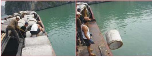
Figure 2. Concrete tanks as artificial reefs are being laid on seabed in Ha Long Bay, North of Vietnam.
