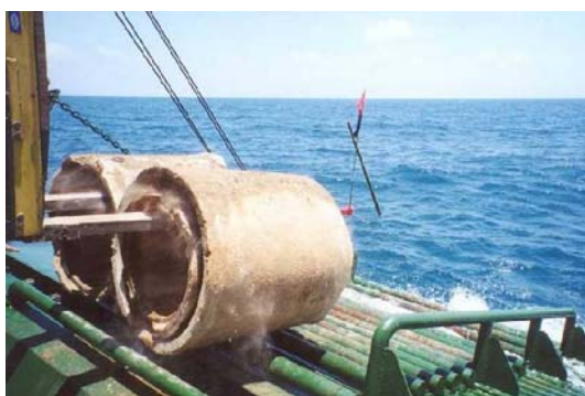
Figure 2c. Materials used for the installation of artificial reef, concrete pipe
