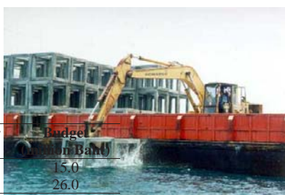
Figure 2b. Materials used for the installation of artificial reef, disc block
