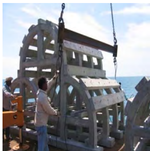
On-board crane lifting the ARs
