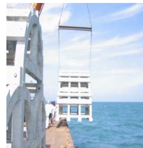
On-board crane lifting the ARs
