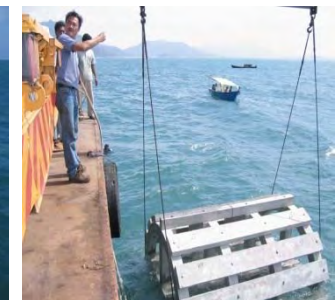
ARs unloaded and placed on the seabed
