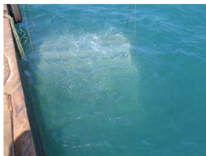
After Unjam Protek is lowered to the seabed, diver's responsibility is to guide the ARs to position in the site
