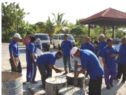
Fig. 6. Preparation of cement anchors
