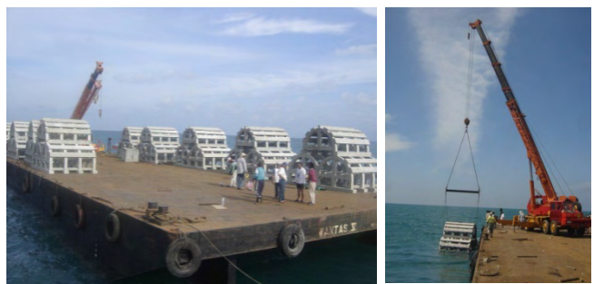
Fig. 31. Installation of ARs by LKIM on 20-22 January 2006
