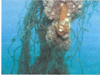
Fig. 35 Marine growth attached on FEDs appendage two month after installation
