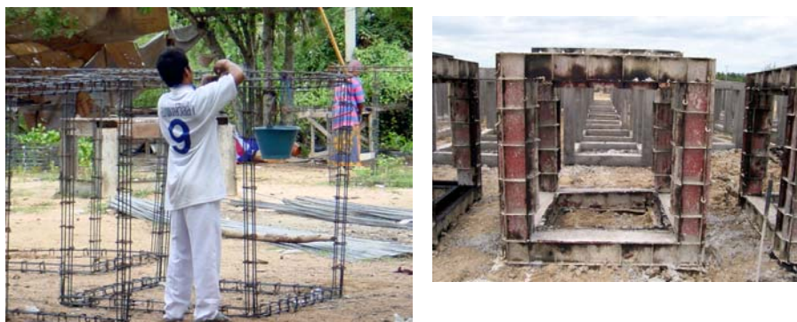
Figure 1. The square concrete tubes with size 2*2*2 m or 1.5*1.5*1.5 m. (Under construction)
