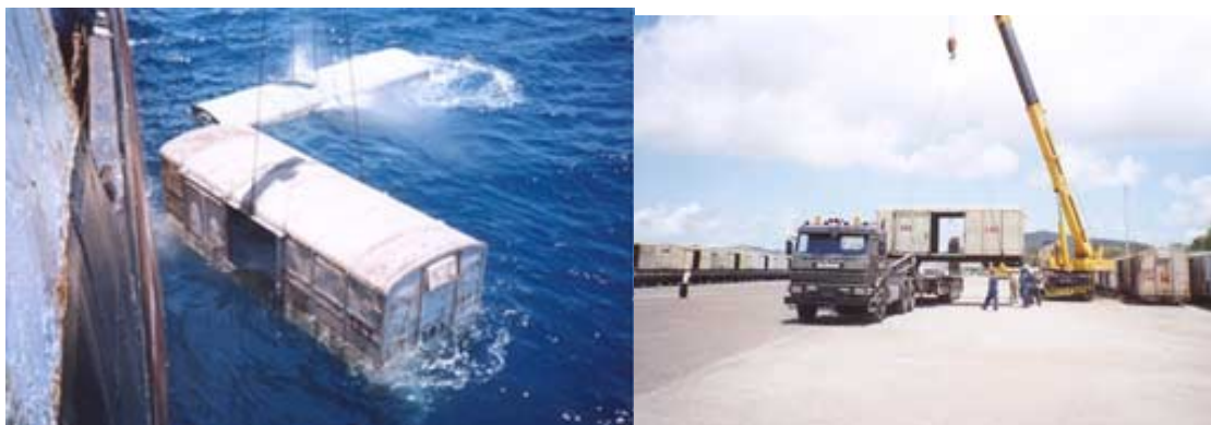
Figure 4. Train wagons used to install artificial reefs
