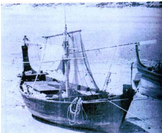
Fig. 6 Squid cast net with light luring
