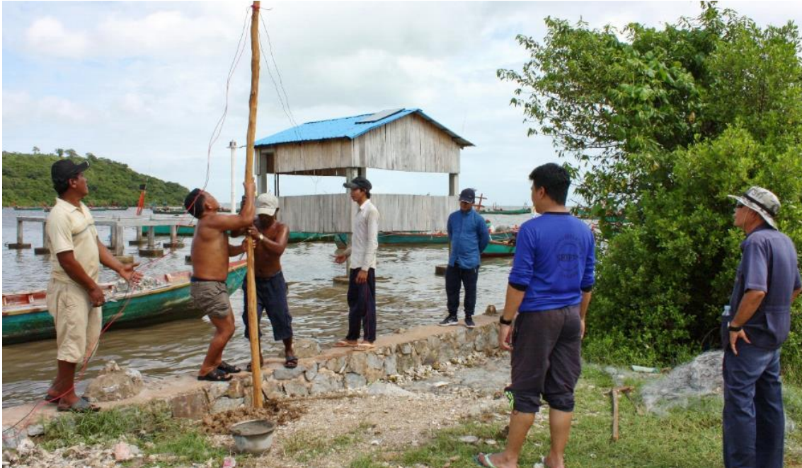
Figure 56. Set-up the electric power system to support crab bank hatchery (August 2019)
