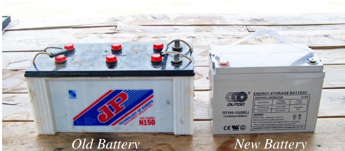
Figure 25. Old battery (left) Replacing with the new battery (Right) (June 2019)
