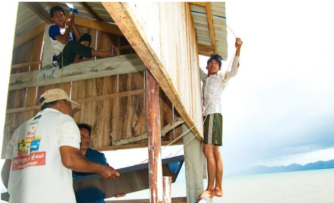
Figure 29. Solar panel system relocating (June 2019)
