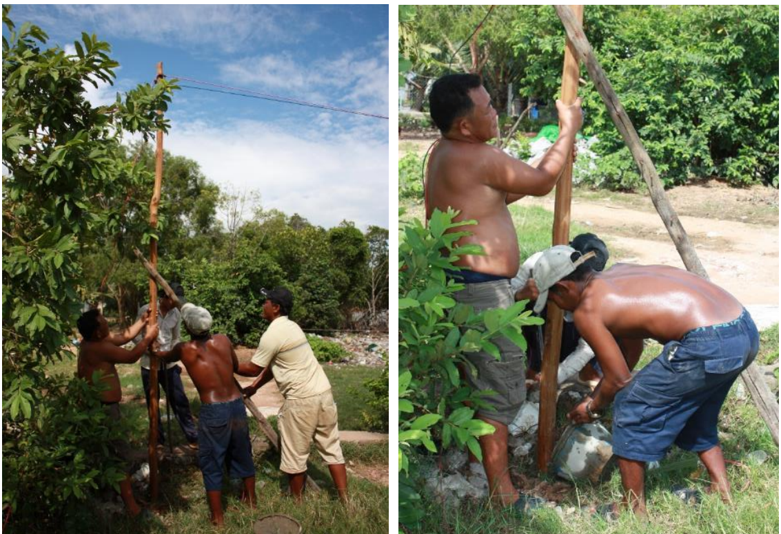
Figure 57. Set-up the electric power system to support crab bank hatchery (August 2019)
