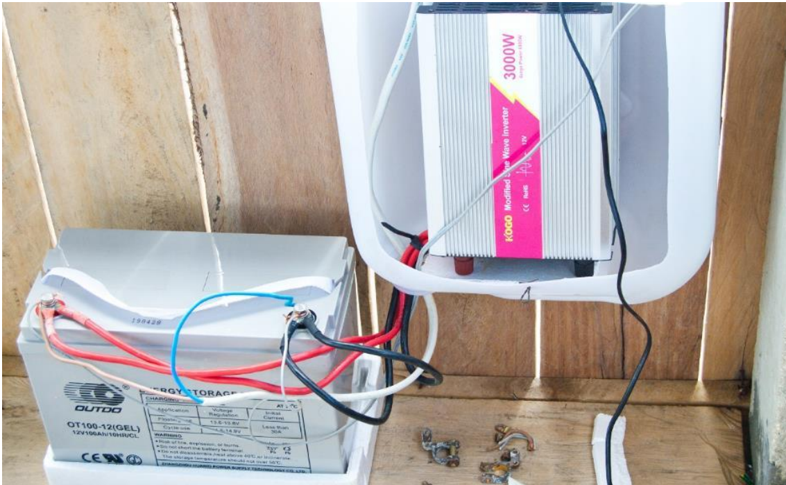
Figure 36. Setting up the new battery and DC/AC power inverter (June 2019)
