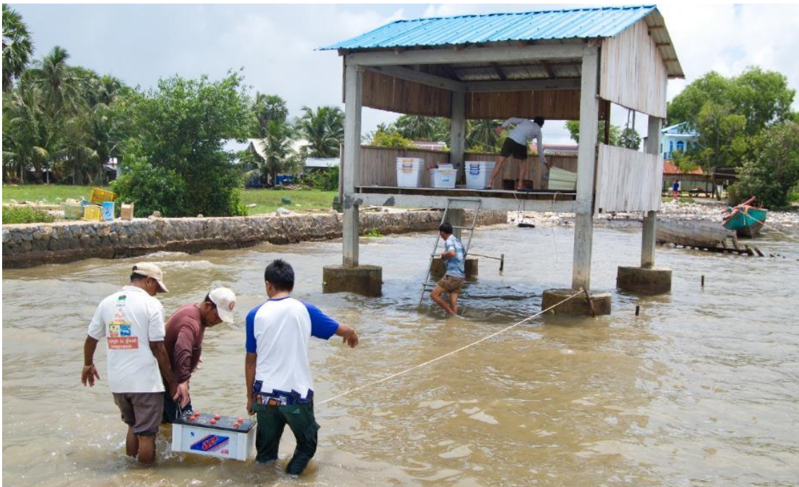
Figure 33. Battery transferring to the new hatchery house (June 2019)
