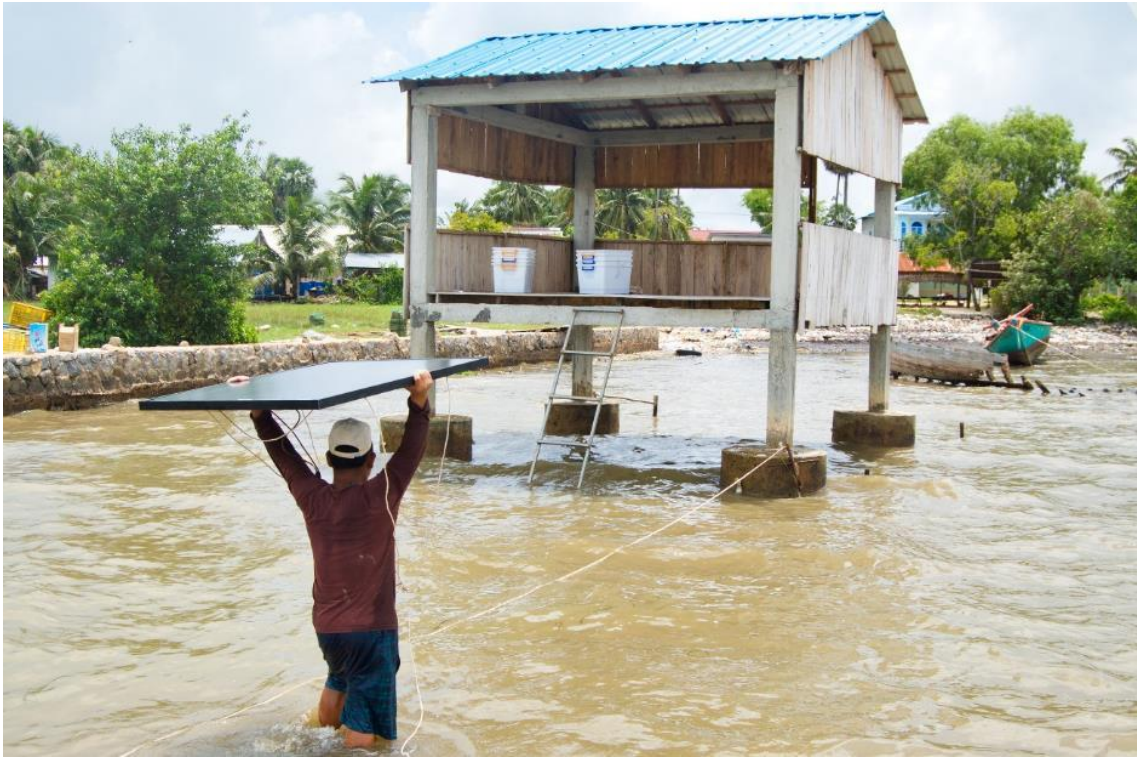
Figure 32. Solar panel transferring to the new hatchery house (June 2019)
