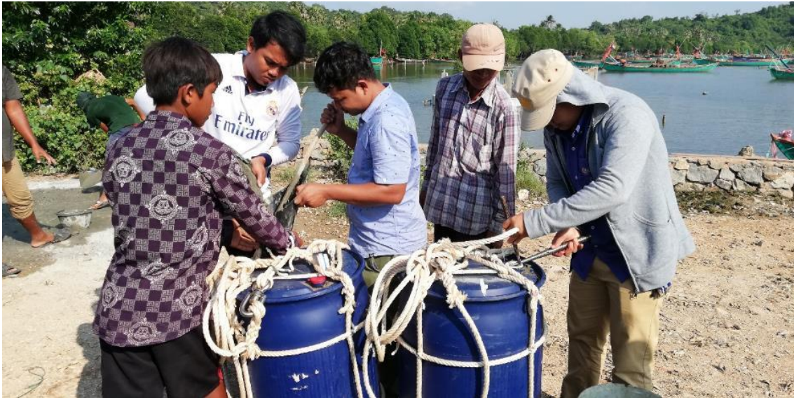
Figure 74. Buoy making (Buoy balancing weight by mixed cement input 2)
