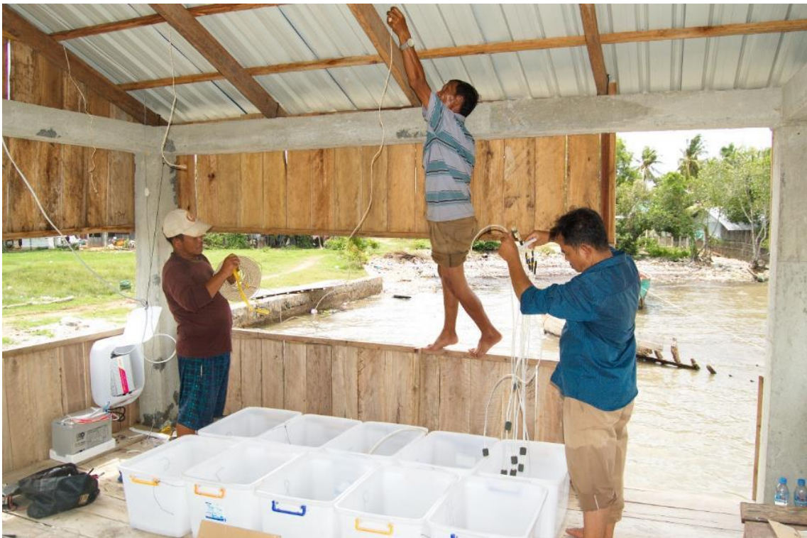
Figure 39. Preparing for the aeration system for each hatching tank containers (June 2019)
