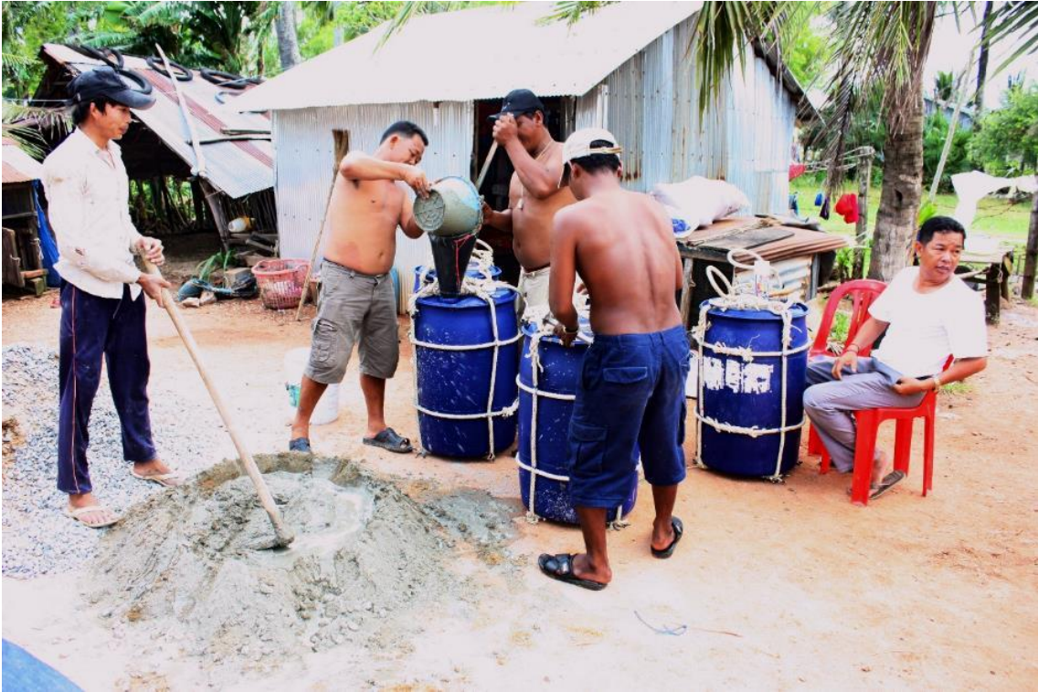
Figure 73. Buoy Making (Buoy balancing weight by mixed cement input 1)
