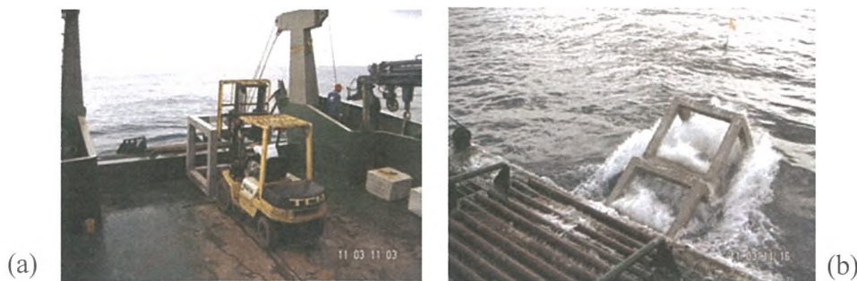
Fig. 6 Fork lift using for convey the cubical shape concrete dumping on the project site (a) the dumping position are marked by anchor flag buoy (b)
