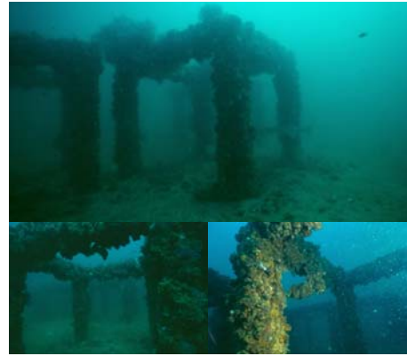
Figure 1. Fouling community on the structures (made of 2x2x2 m open concrete cubes) of AR in Ranong Province about 3 years after installation.
